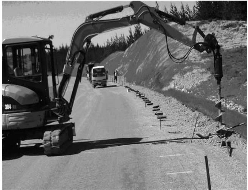
Guardrail installation
