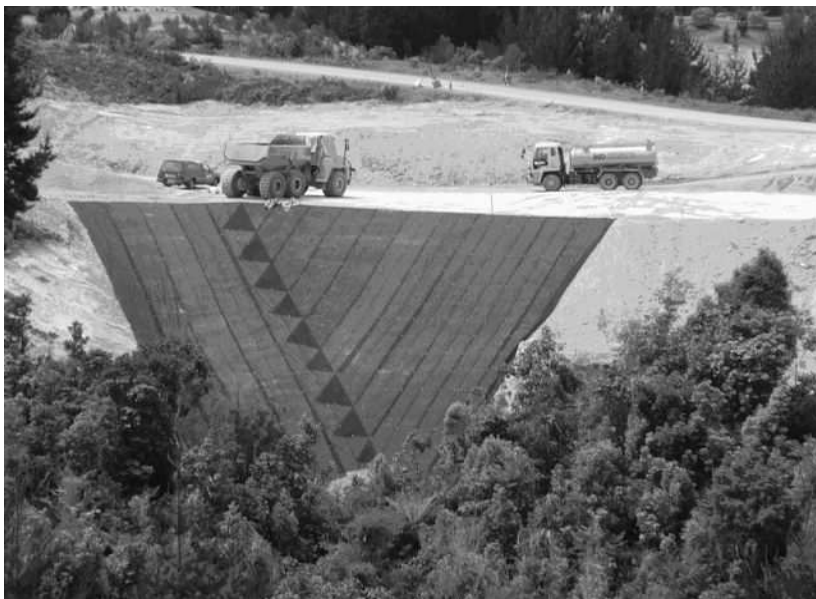
Enkamat placed on batter by Chaytor Road
