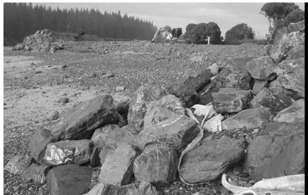
After a series of swells, the rock wall was partially demolished by the force of the sea. This photo was taken in mid-August 2009. Dune Trust member Jim Dahm said that dune areas close to large estuaries like this are often subject to greater movement of sand and erosion than dune areas on ordinary beachfronts.
