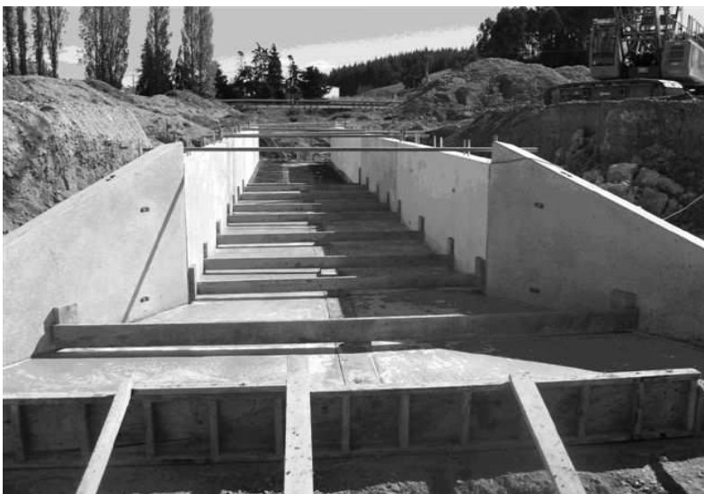
Early work on the Higgs single box culvert
