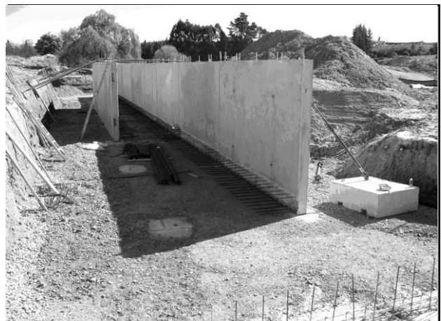
Dominion culvert construction.
