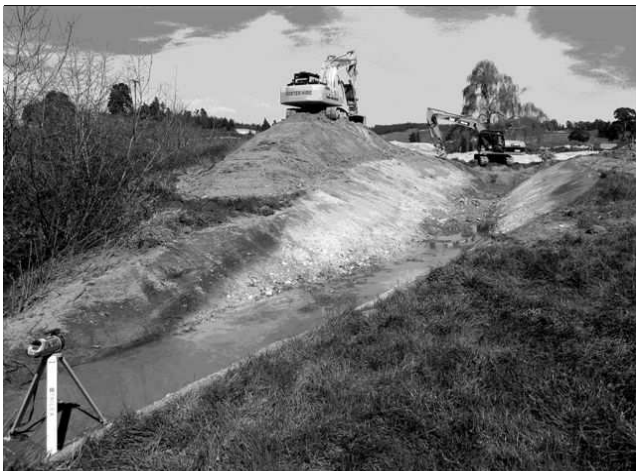
Field Creek diversion excavation.
