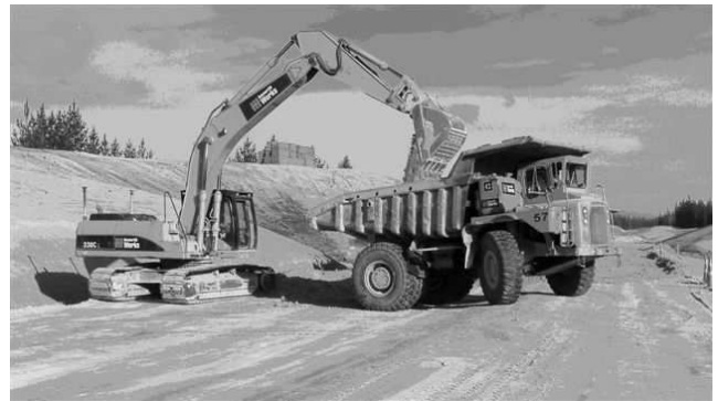
Undercutting of sub-base through forest corridor
