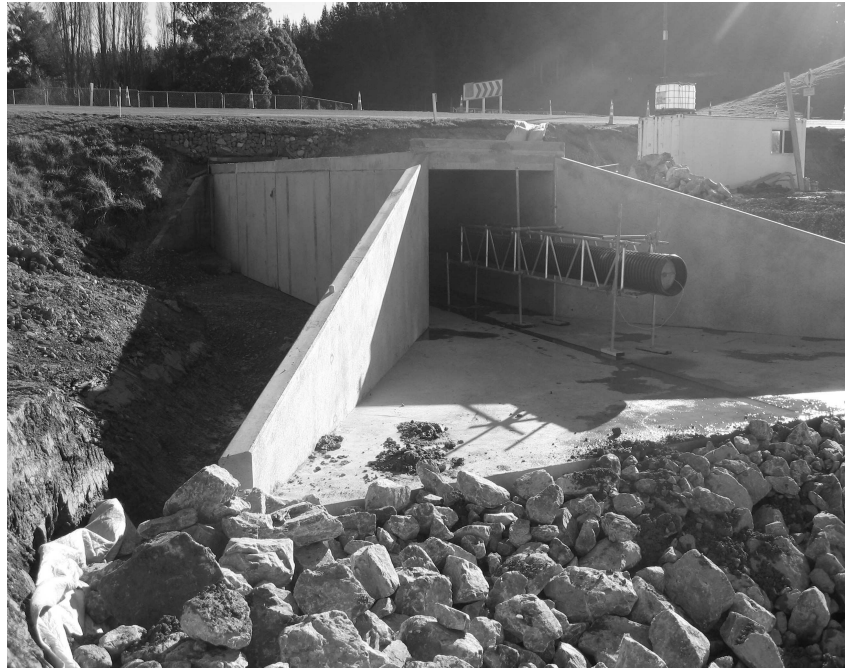
Trafalgar Road culvert
